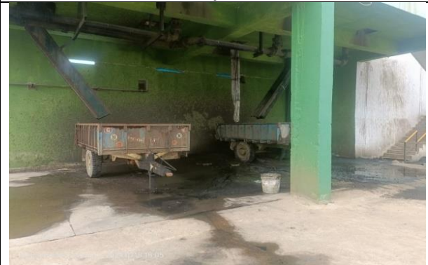
Collection of sludge in trolley
